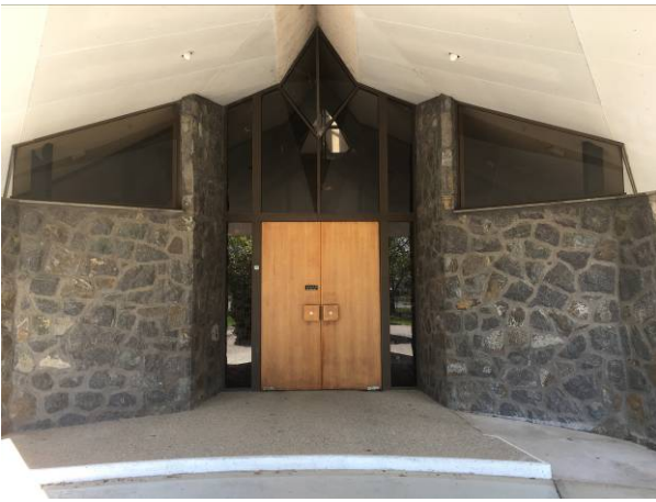
Image 7 Port-Cochere. Main entrance (ACT Heritage 2016)
