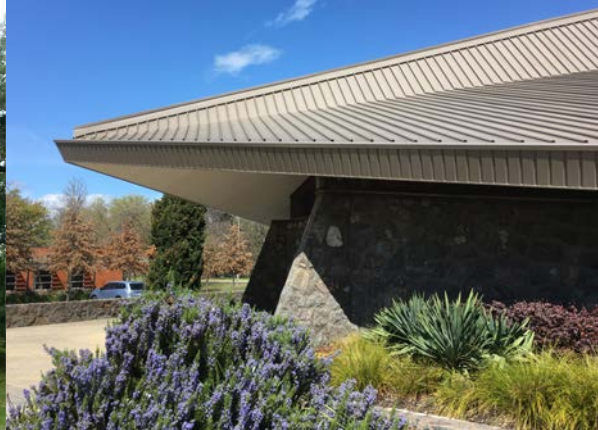
Image 15 Roofline at St Joseph's (ACT Heritage 2016)
