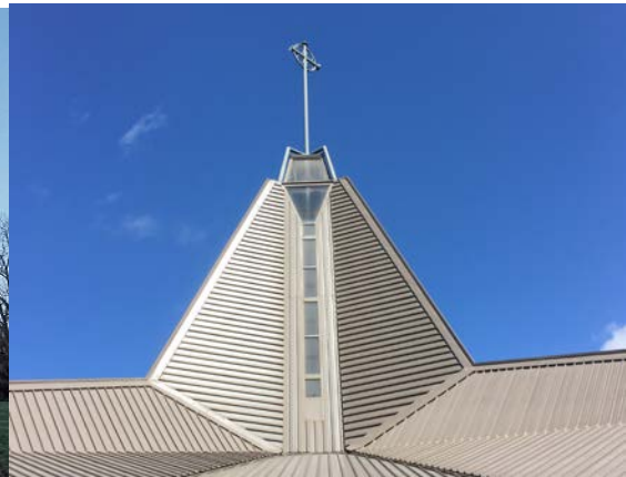
Image 17 Tower at St Joseph's (ACT Heritage 2016)
