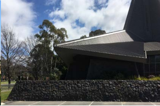
Image 13 St Joseph's roof (ACT Heritage 2016)
